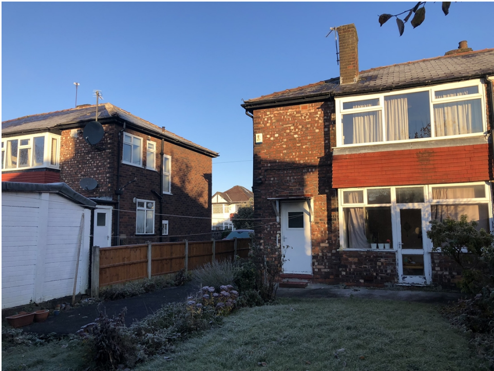
Figure 3. Rear view of property as seen from the applicant's rear garden.
